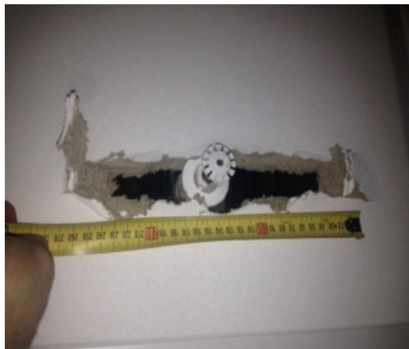
Figure 10: Relative movement of sprinkler and ceiling
